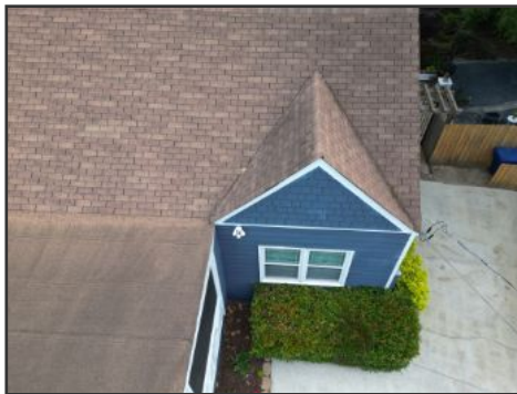
DJI drone image of roof covering
