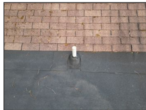
example vent penetration
