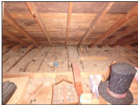
general image of attic / roof framing
