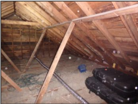
general image of attic / roof framing
