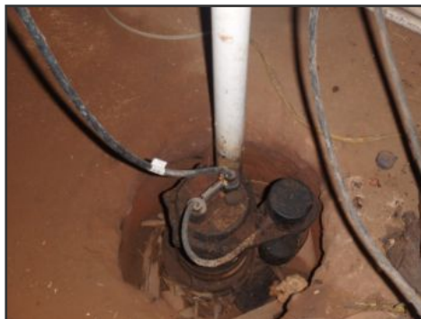
sump pump condition
