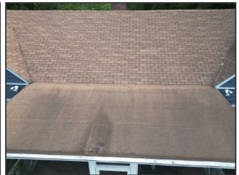
DJI drone image of roof covering
