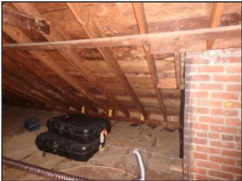
general image of attic / roof framing
