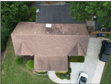
DJI drone image of roof covering
