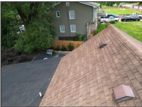
DJI drone image of roof covering
