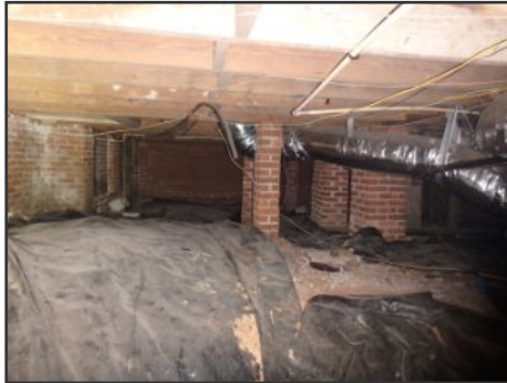
general image of crawl space
