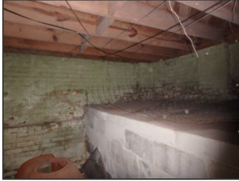
general image of crawl space
