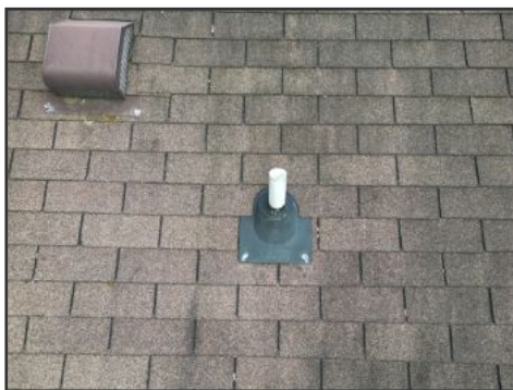
example vent penetration
