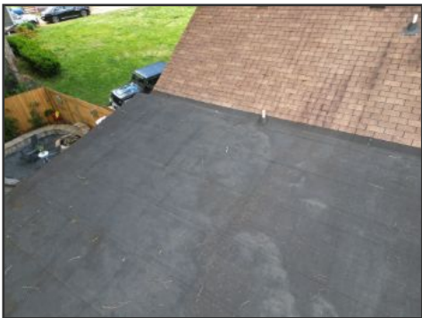
DJI drone image of roof covering
