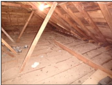
general image of attic / roof framing
