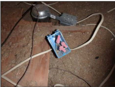
improper junction--attic
