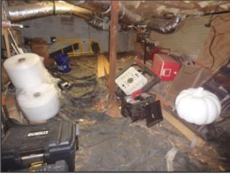
general image of crawl space
