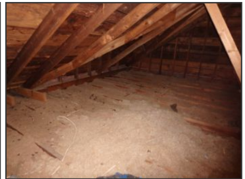
general image of attic / roof framing
