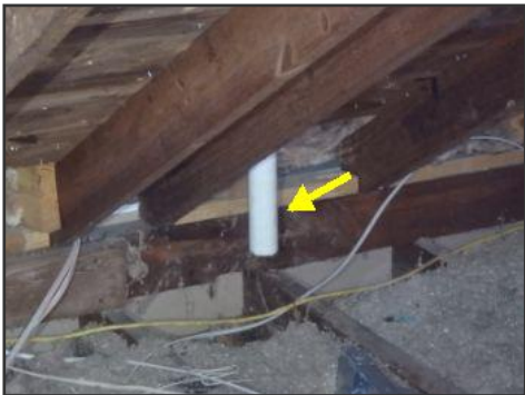
unused PVC vent pipe
