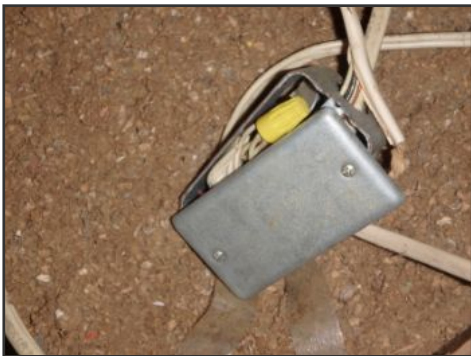
improper junction--attic
