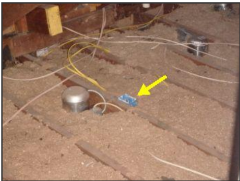
improper junction--attic
