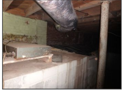
general image of crawl space
