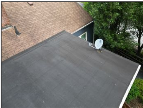
DJI drone image of roof covering
