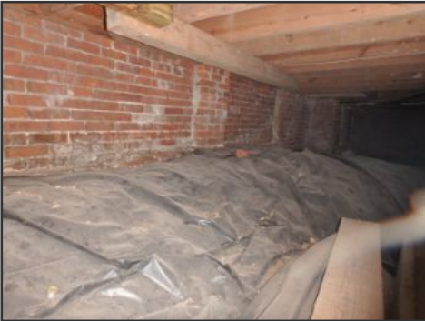
general image of crawl space
