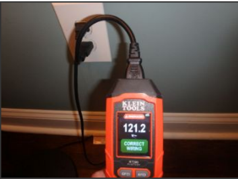
example receptacle testing
