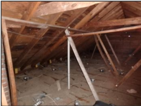
general image of attic / roof framing
