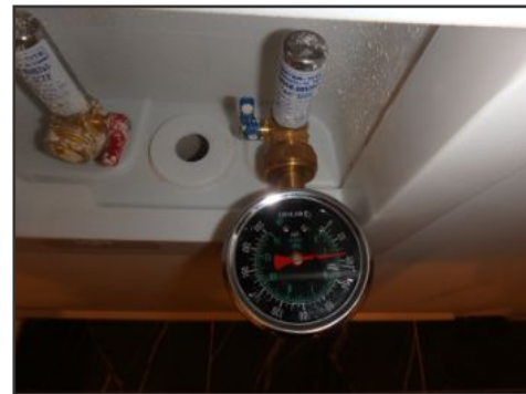
water pressure test
