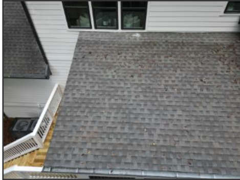
DJI drone image of roof covering
