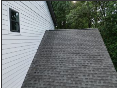
DJI drone image of roof covering
