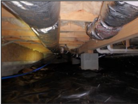
general image of crawl space
