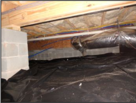
general image of crawl space
