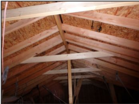
general image of attic / roof structure
