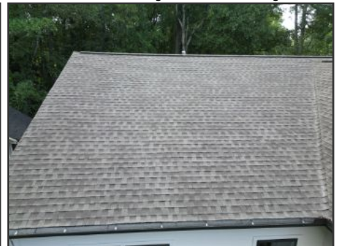
DJI drone image of roof covering
