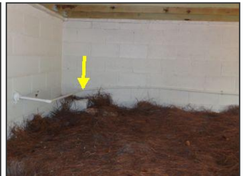
"valley" at condensation drain pipe
