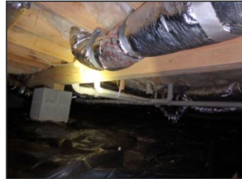
general image of crawl space
