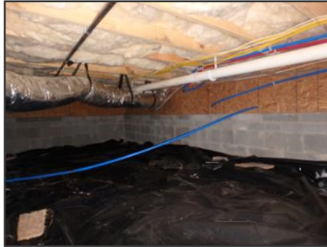
general image of crawl space
