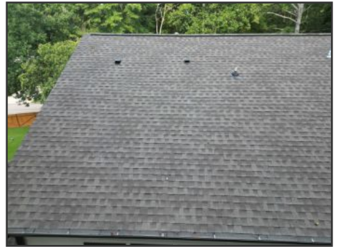
DJI drone image of roof covering
