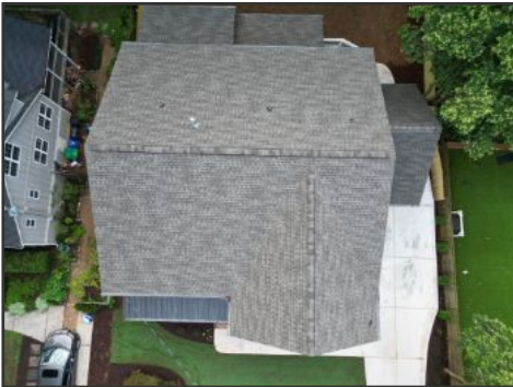
DJI drone image of roof covering
