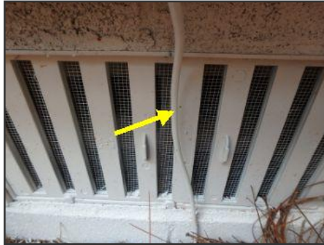
grounding conductor
