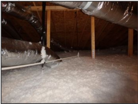
general image of attic / roof structure
