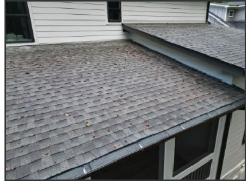
DJI drone image of roof covering
