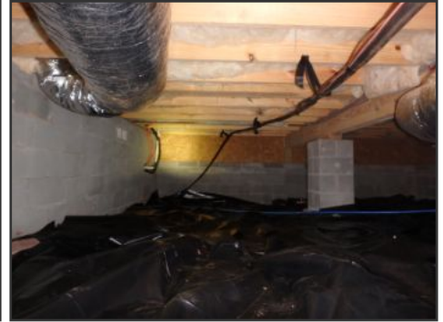
general image of crawl space
