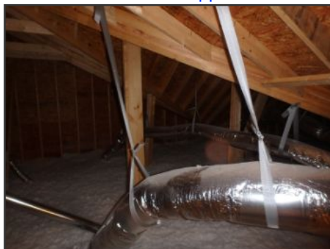
general image of attic / roof structure
