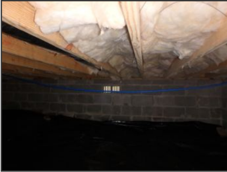
general image of crawl space
