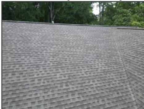
DJI drone image of roof covering
