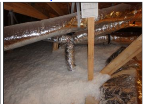
general image of attic / roof structure
