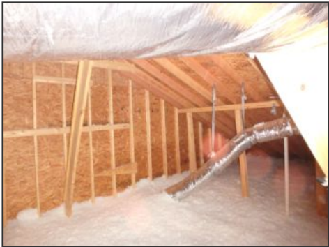
general image of attic / roof structure
