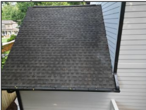
DJI drone image of roof covering
