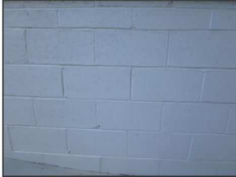
example foundation wall condition
