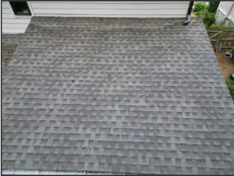
DJI drone image of roof covering
