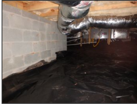
general image of crawl space
