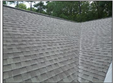
DJI drone image of roof covering
