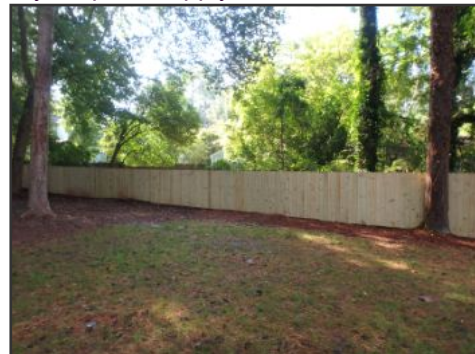
example fence condition
