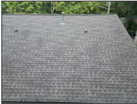
DJI drone image of roof covering
