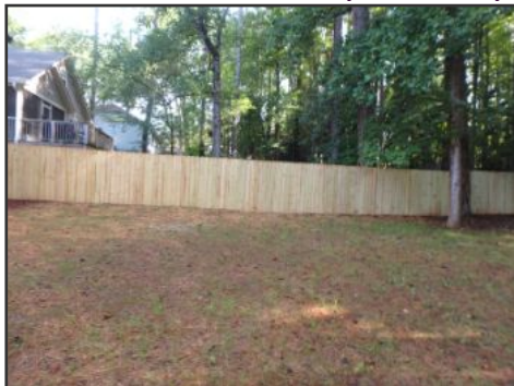
example fence condition
