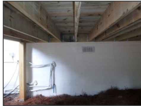
underside of deck
