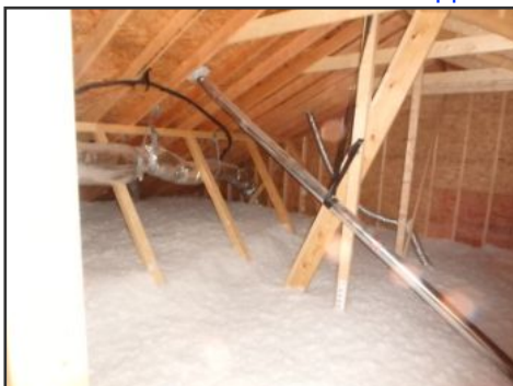
general image of attic / roof structure
