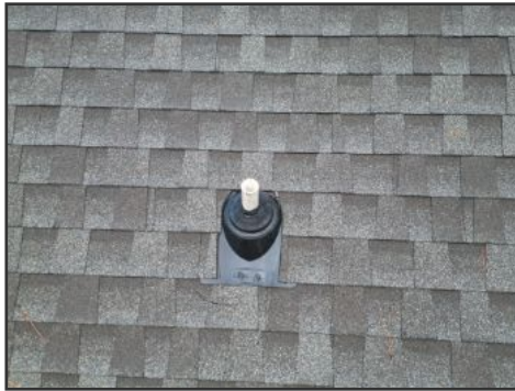
example plumbing vent penetration
