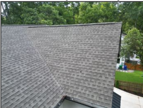
DJI drone image of roof covering
