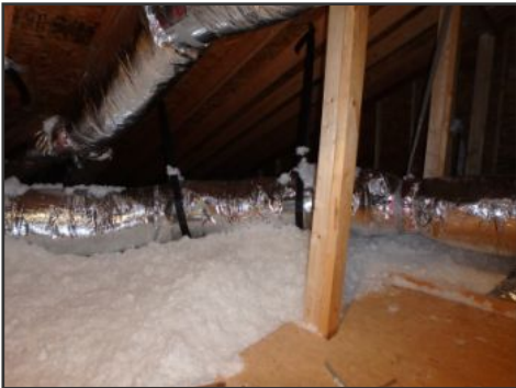
general image of attic / roof structure
