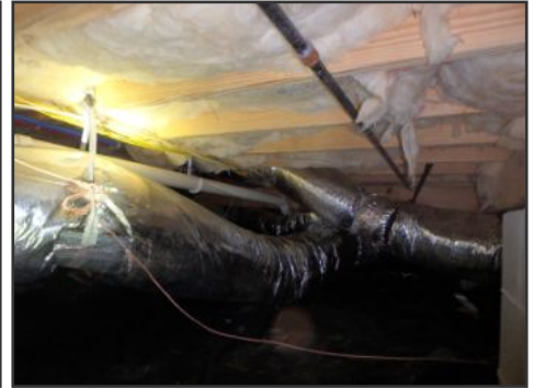
general image of crawl space
