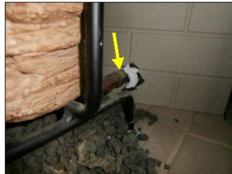
*proper sealant should be installed*
