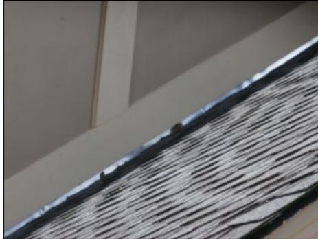
*no visible step flashing*
