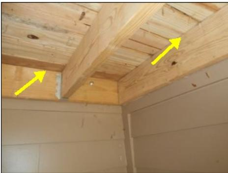
no visible flashing at deck attachment
